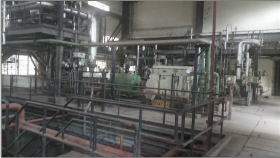
Condition of HP Boiler Feed Pumps
