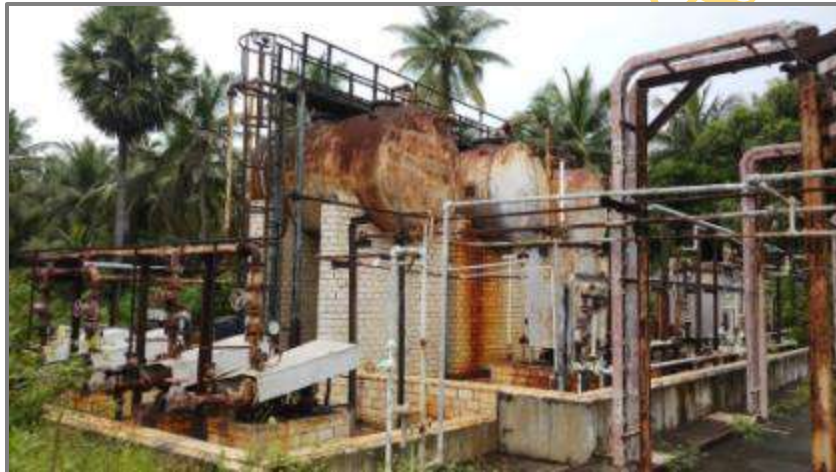
Tanks for DM plant
