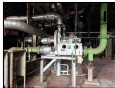
Gland Steam Condenser & Name Plate
