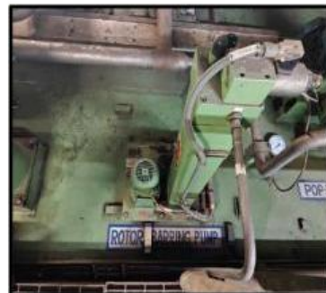
Rotor Barring Pump
