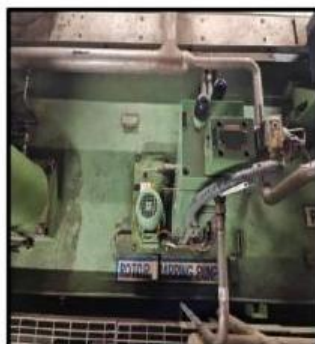
Rotor Barring Pump
