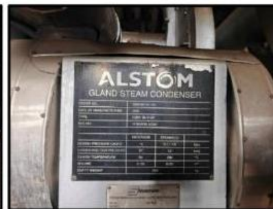
Gland Steam Condenser & Name Plate
