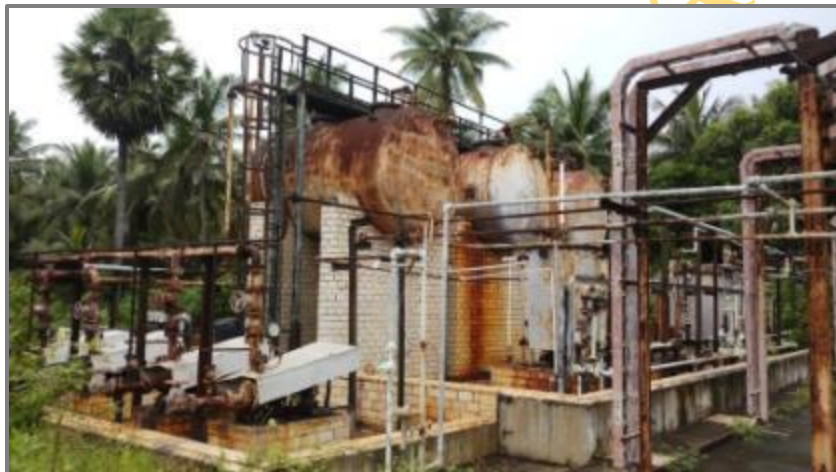
Tanks for DM plant
